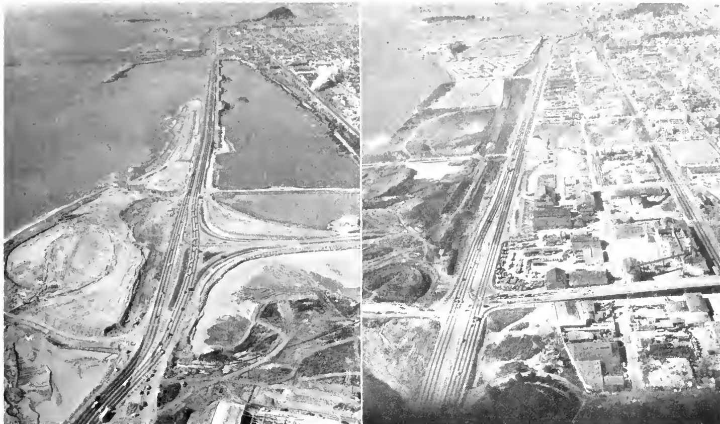
LEFT: Some idea of amount of dredger fill required for new Ashby Avenue interchange may be gleaned from this picture. Hydraulic fill will be shaped to provide roadways for trumpet loop of new interchange. Hydraulic fill is being placed at lower right of picture from a pipe line, visible in foreground, passing under existing highway. RIGHT: View of northerly portion of project with University Avenue intersection in foreground and El Cerrito overhead, northerly terminus of project, in background. Excavation to left of existing highway results from removal of some 400,000 cubic yards of unsuitable material prior to placement of hydraulic sand fill.
